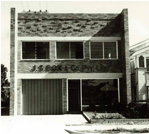
THE FIRST BOX HEADQUARTERS, 1943.
